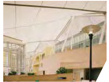
Tensile Structures / Fabric Roofing
